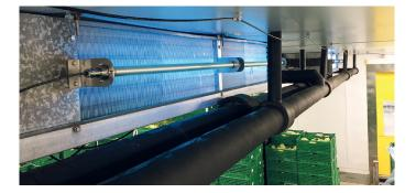
sterilAir<sup>®</sup> offers a powerful and environmentally friendly solution. Our UVC installations sustainably prevent build up and growth of biofilm. Clean coils keep energy consumption of the cooling unit constantly low. The slats remain hygienically flawless, cleaning effort and frequency decrease significantly - a considerable cost saving in operation and maintenance.
